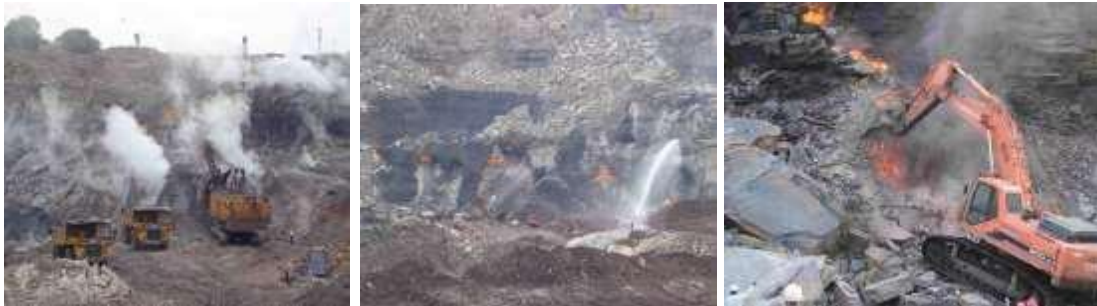
Fire excavation at Muraidih Fire excavation at Bararee
