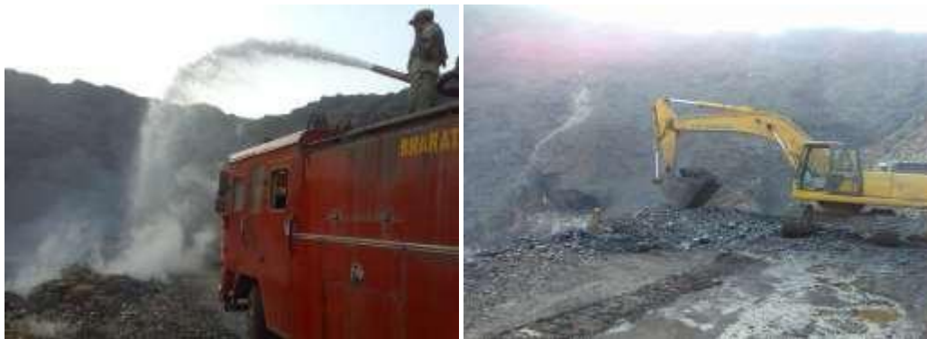
Fire excavation at Ena OC
