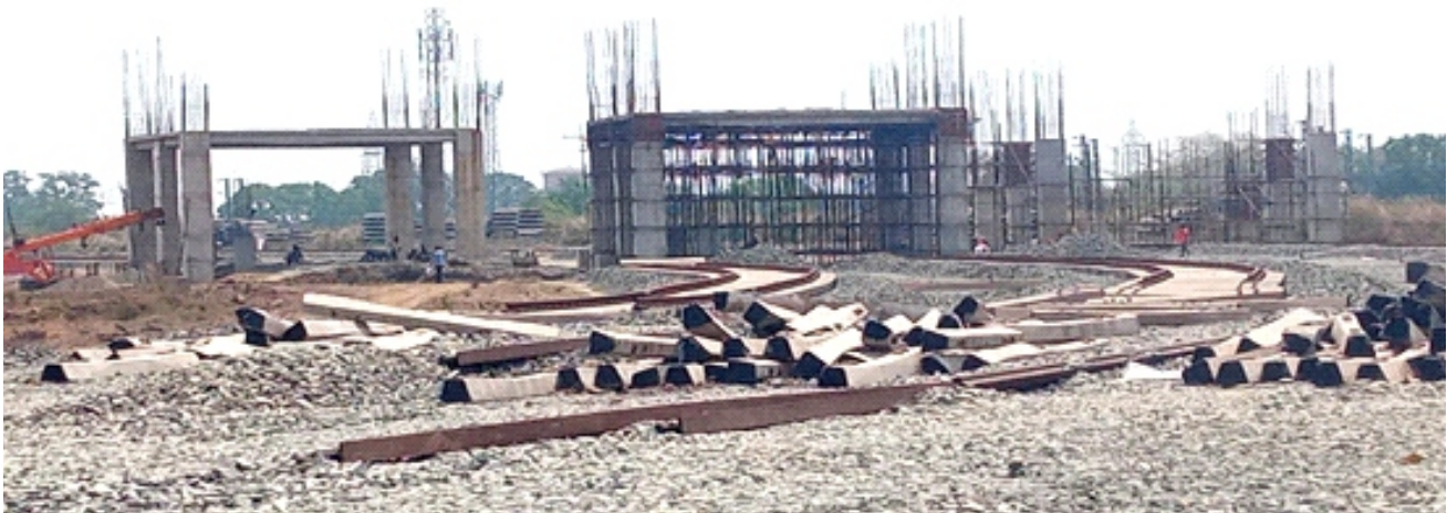
2.5 Mtpa Patherdih NLW WASHERY UNDER CONSTRUCTION
