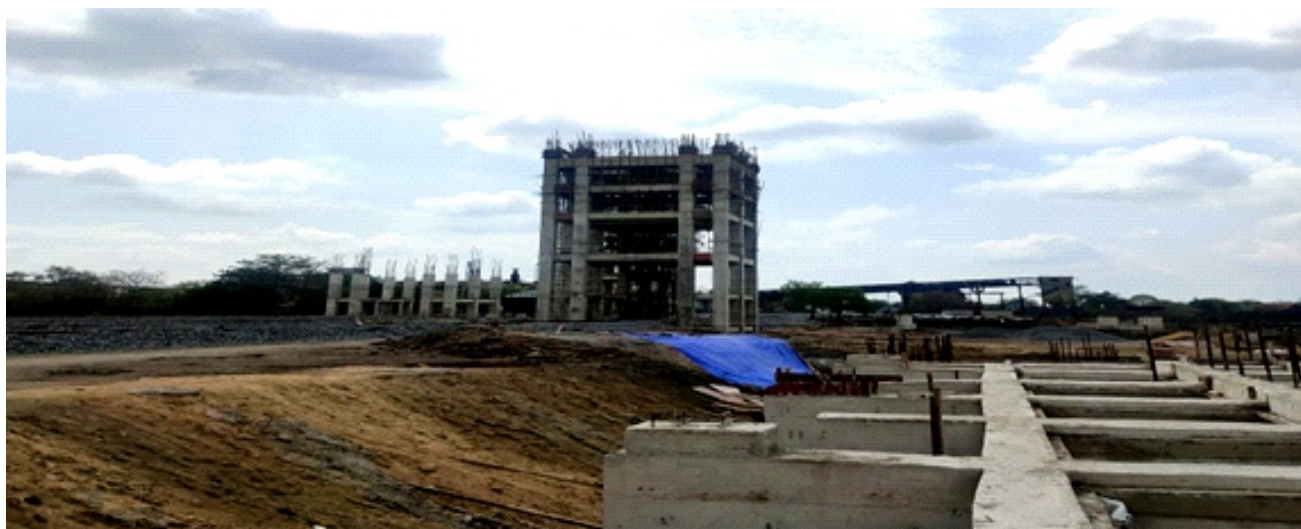
2.0 MTPA BHOJUDIH NLW WASHERY UNDER CONSTRUCTION
