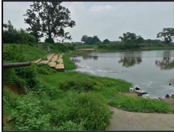
Pond Constructed for Villagers at KB 10/12 Colliery
