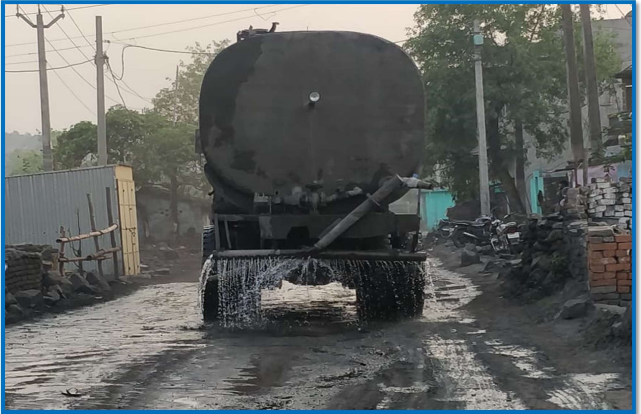
Picture 4 (I) – Water Sprinkling on Transportation Road
