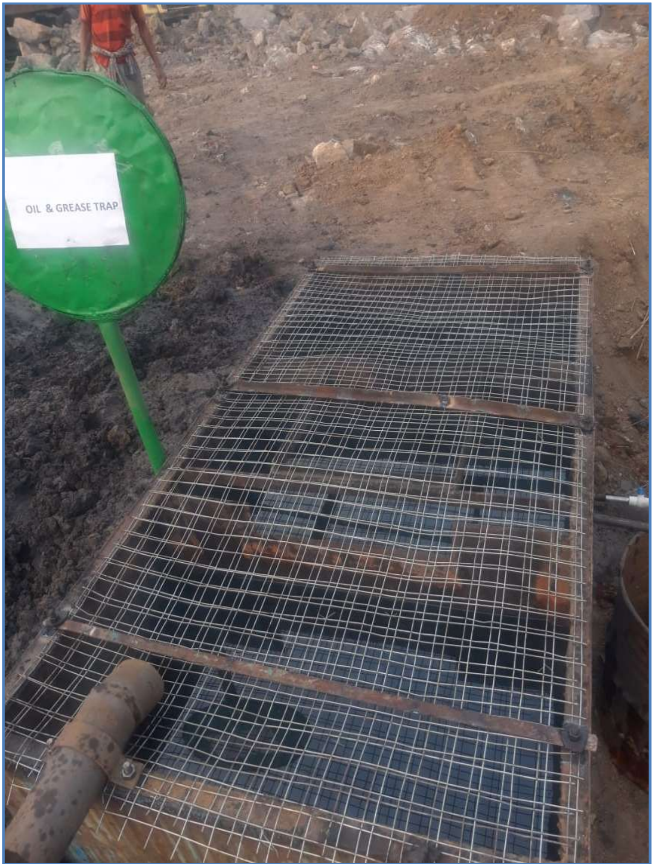
Picture 7 – Oil & Grease Trap
