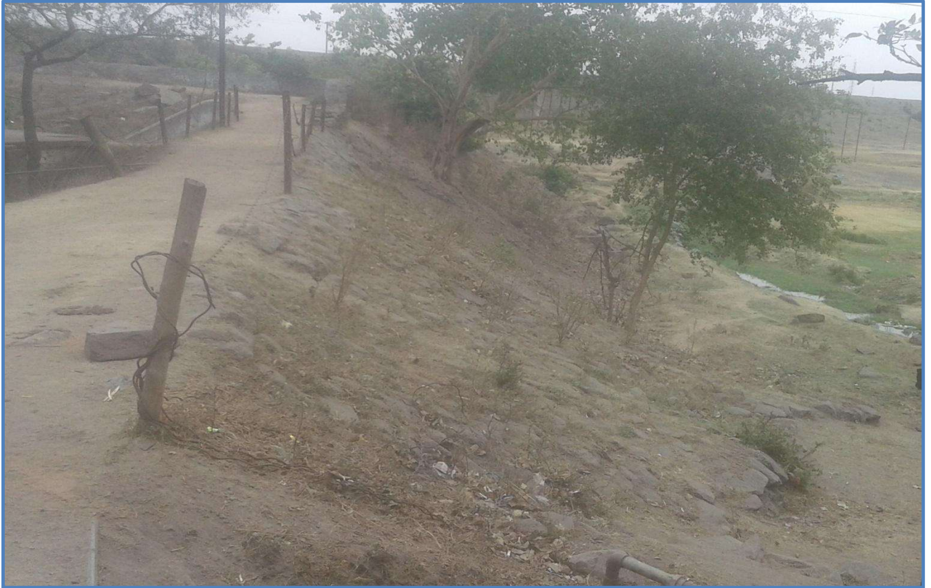
Picture 5 - Stone Pitching/embankment at Kari Jore
