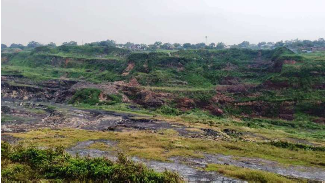
Figure 19: Subsidence area in Bagdigi Mines
