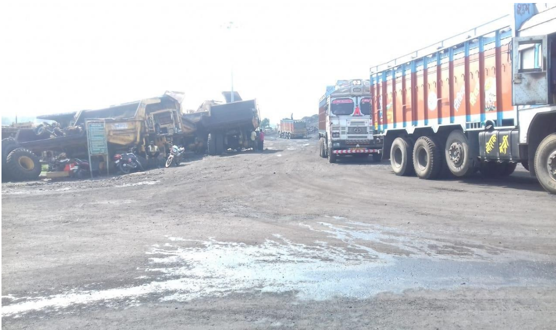
Roads constructed within colliery premises
