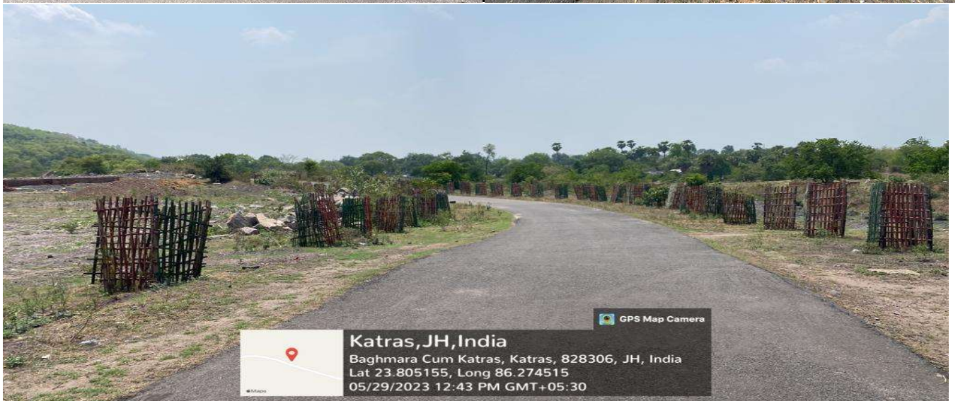
Bamboo gabion plantations along roads.
